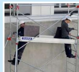
**INSTALLATION EN SÉCURITÉ DU PLANCHER**
